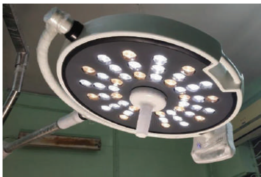
Solitaire 48 Ceiling Installation at Andhra Pradesh, India
