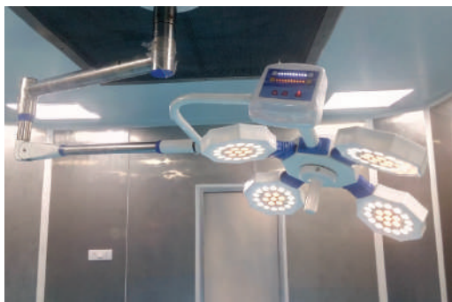
Star 84 Ceiling Installation at Earth Hospital (Gujarat, India)
